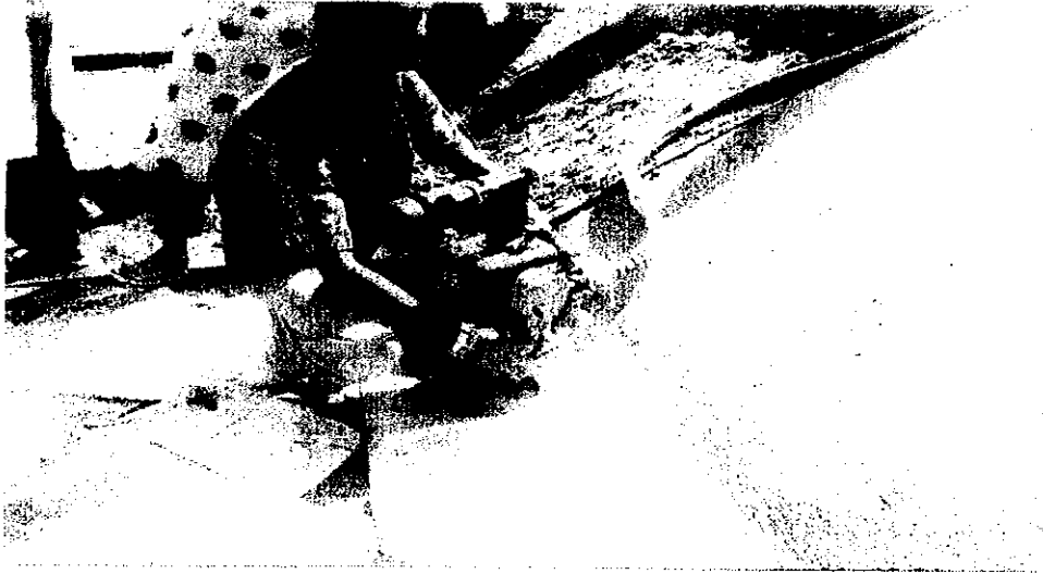
1. DIESEL OPERATED NEEDLE VIBRATOR
